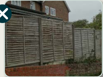
High, non-permeable slatted timber fencing fronting the pavement.
