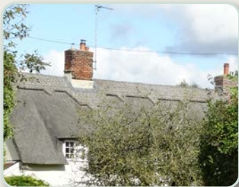
Thatched roof with red brick chimney stack
