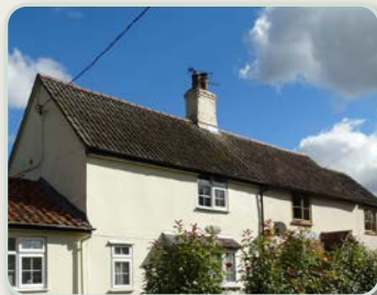
Brown clay tile pitched roof with chimney stack
