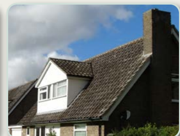
Brown gabled clay tile roof with dormer and external chimney breast
