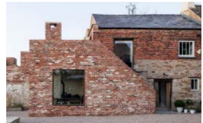
Figure 54: Recycled and reclaimed bricks used for an extension to a traditional dwelling in Gretton, UK.
